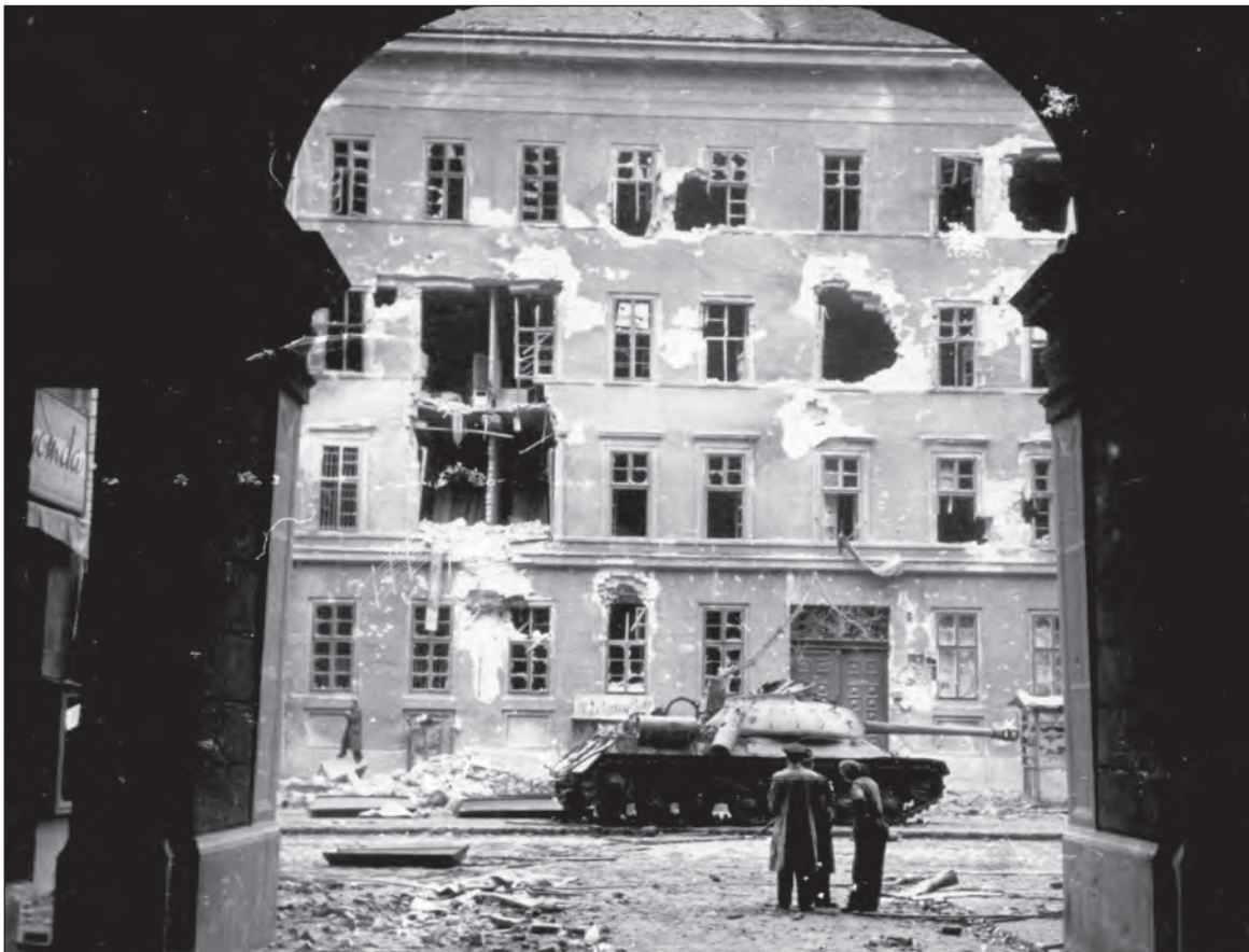
The tunnel between the Corvin Movie Theater and Kilián Barracks
