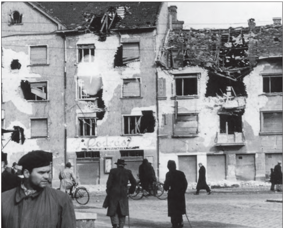
Damage from the Revolution
