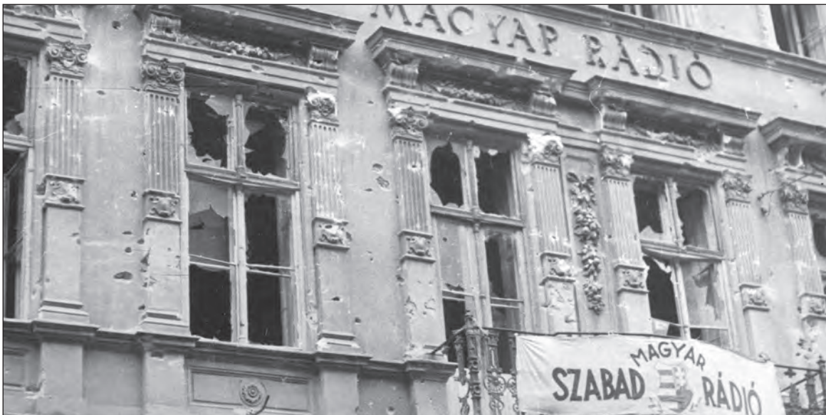
The damaged facade of the Hungarian Radio building after freedom fighters hung a new banner reading "Free Hungarian Radio"
